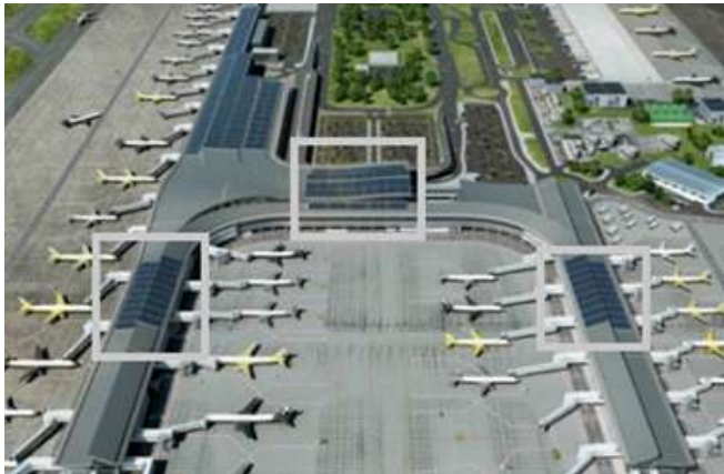
Figure 6. El Dorado Airport Solar Panels, Terminal 1. [12]
