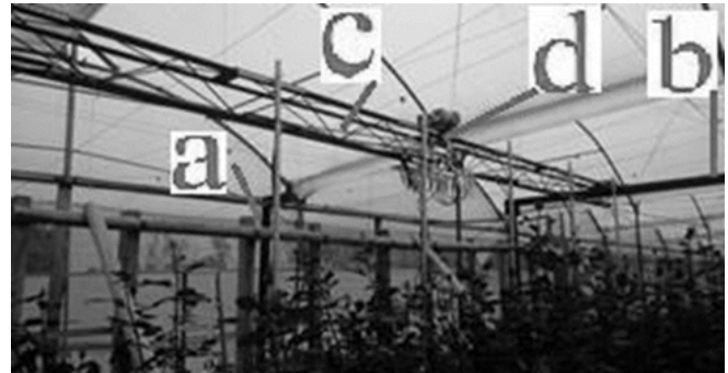
Figure 3. Mobile carriage and support structure of the booms mounted on the travel rails. Source: own.
