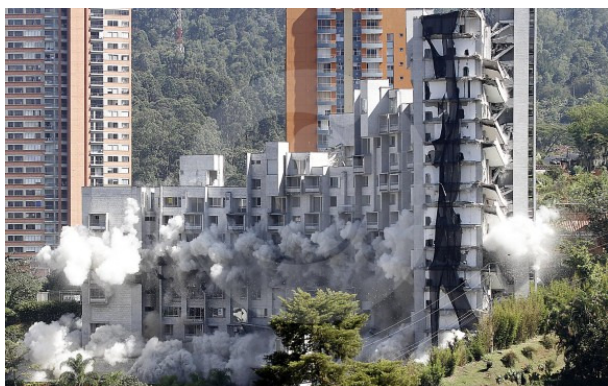
Figure 11. Demolition of towers 1, 2, 3, 4 and 5 (Mercado, 2019).
