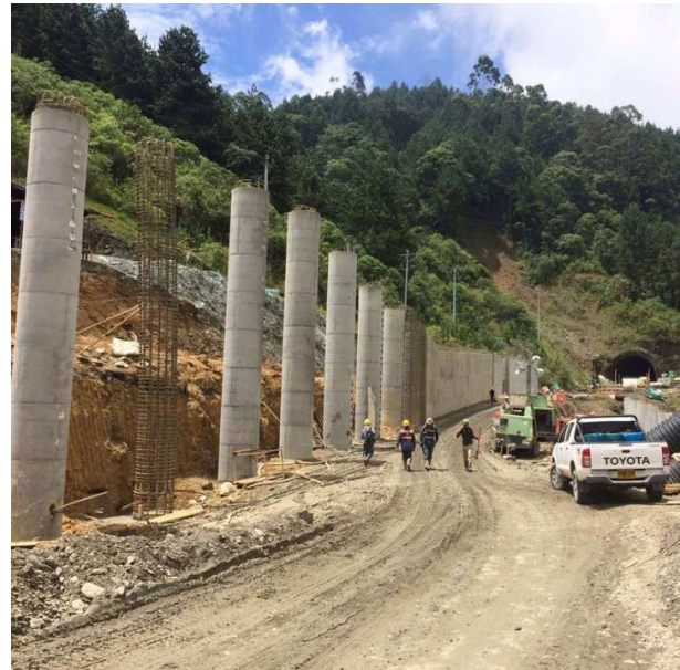
Figure 6. Works attached to the tunnel (Icconstructores, 2017).
