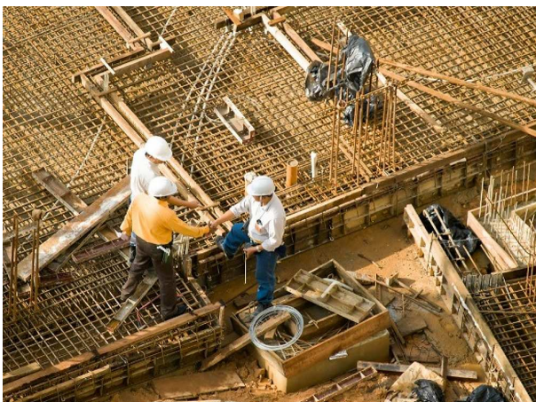
Figure 1. Civil works (Group, 2017).
