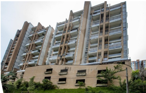
Figure 12. Continental Tower photo, October 2018 (Sánchez, 2019).
