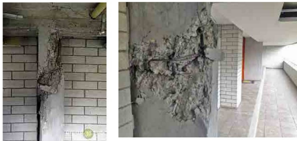
Figure 8. Photographs of the columns before collapse (Suárez, 2019).
