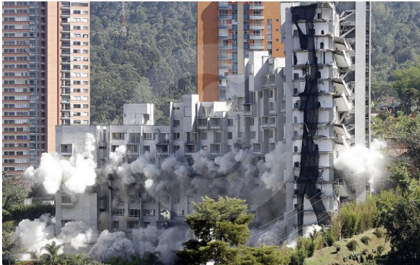
Figure 11. Demolition of towers 1, 2, 3, 4 and 5 (Mercado, 2019).
