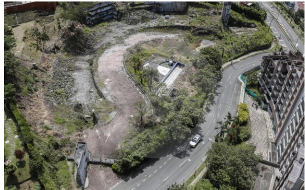
Figure 13. Lot of the Space building after demolition (Sáenz, 2019).
