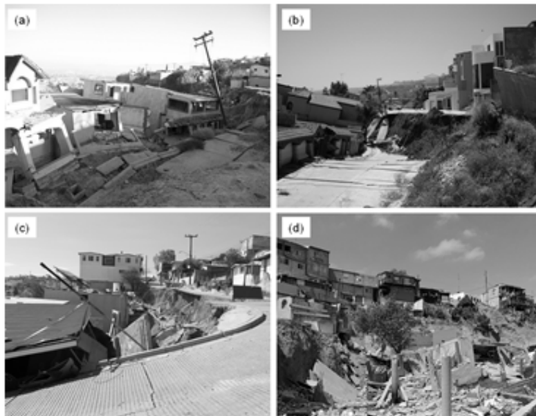
Figure 1. Some urban landslides occurred in Tijuana.
